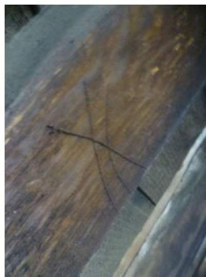
Photo 4: One of the builder's marks on a rafter
