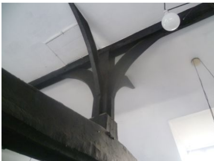
Photo 3: Moulded crown post, with four up-braces.
