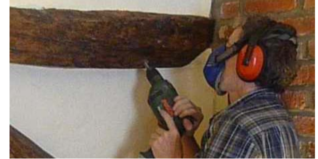
Core extraction in progress.
