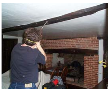
Photo 3: Extraction of a core in progress
