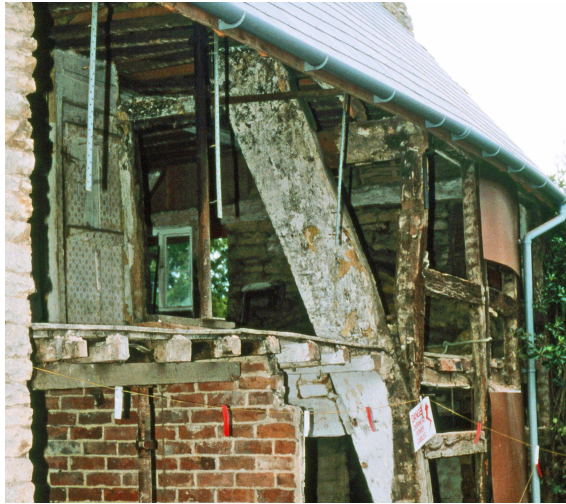
Fig. 4. The cruck construction of Shady Nook in Gotherington was exposed in 1979 when the building was extensively renovated
